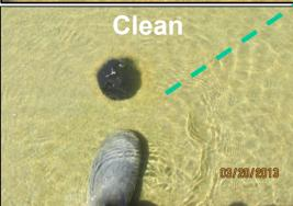
The DeCordova Bend Dam hearth has hundreds of 4-inch drain holes spaced throughout the concrete slabs of the Hearth Sill. The drain holes help relieve uplift pressure. Due to their location in the hearth below the spillway, the drain holes regularly collect debris and are very difficult to keep clean.
